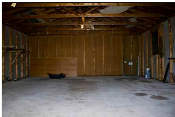
Interior of barn
