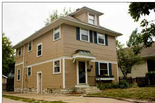
Front Driveway View
